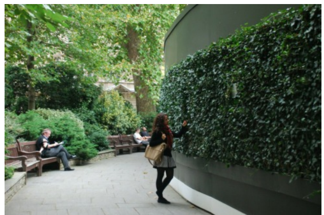
Ivy screen for a building site
